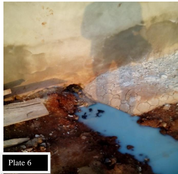
Plate 6: Drain emptied to the Road
