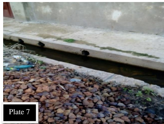
Plate 7: Inadequate Drain
