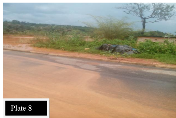
Plate 8: Building on Flood Channel/Road without Drainage
